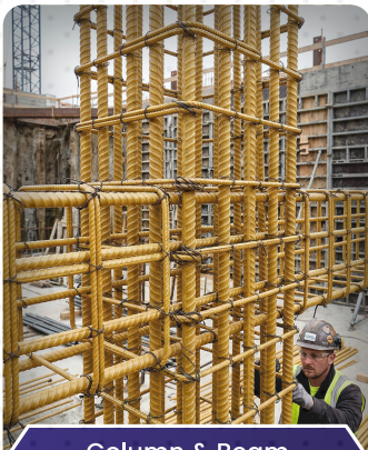
Column & Beam Reinforcement
