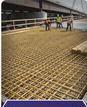
Bridge Deck Construction
